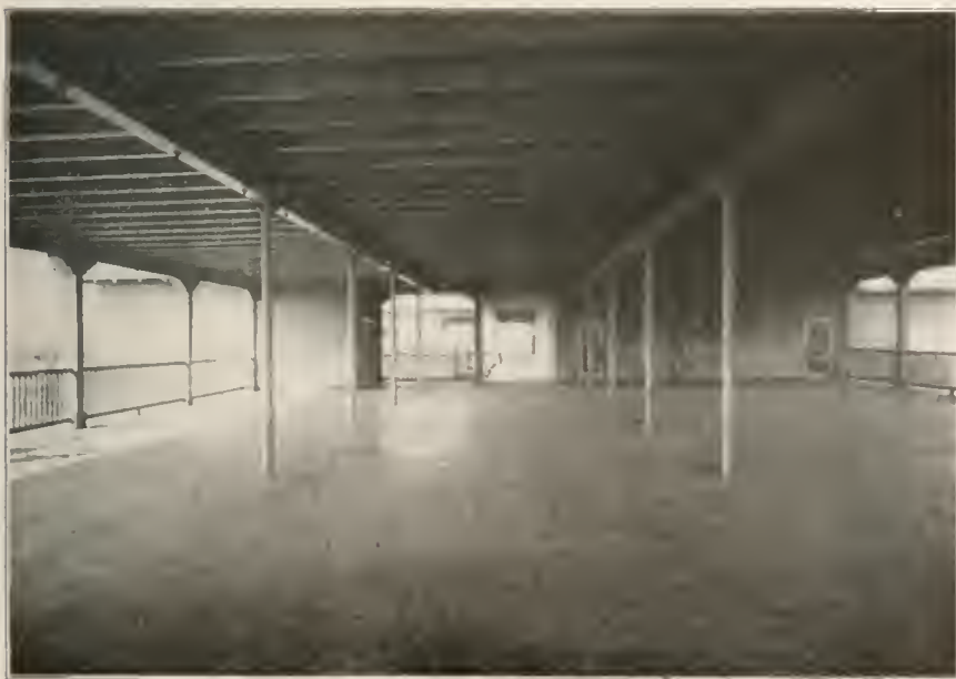
Covered roof gymnasiums, equipped with toilets and drinking fountains, constitute an aid to all varieties of open air activities with children. The floor of this one is covered with battleship linoleum.
